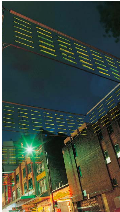
Sussex Street lights, by McGregor Westlake Architecture, provide a cultural overlay Photo: McGregor Westlake Architecture
